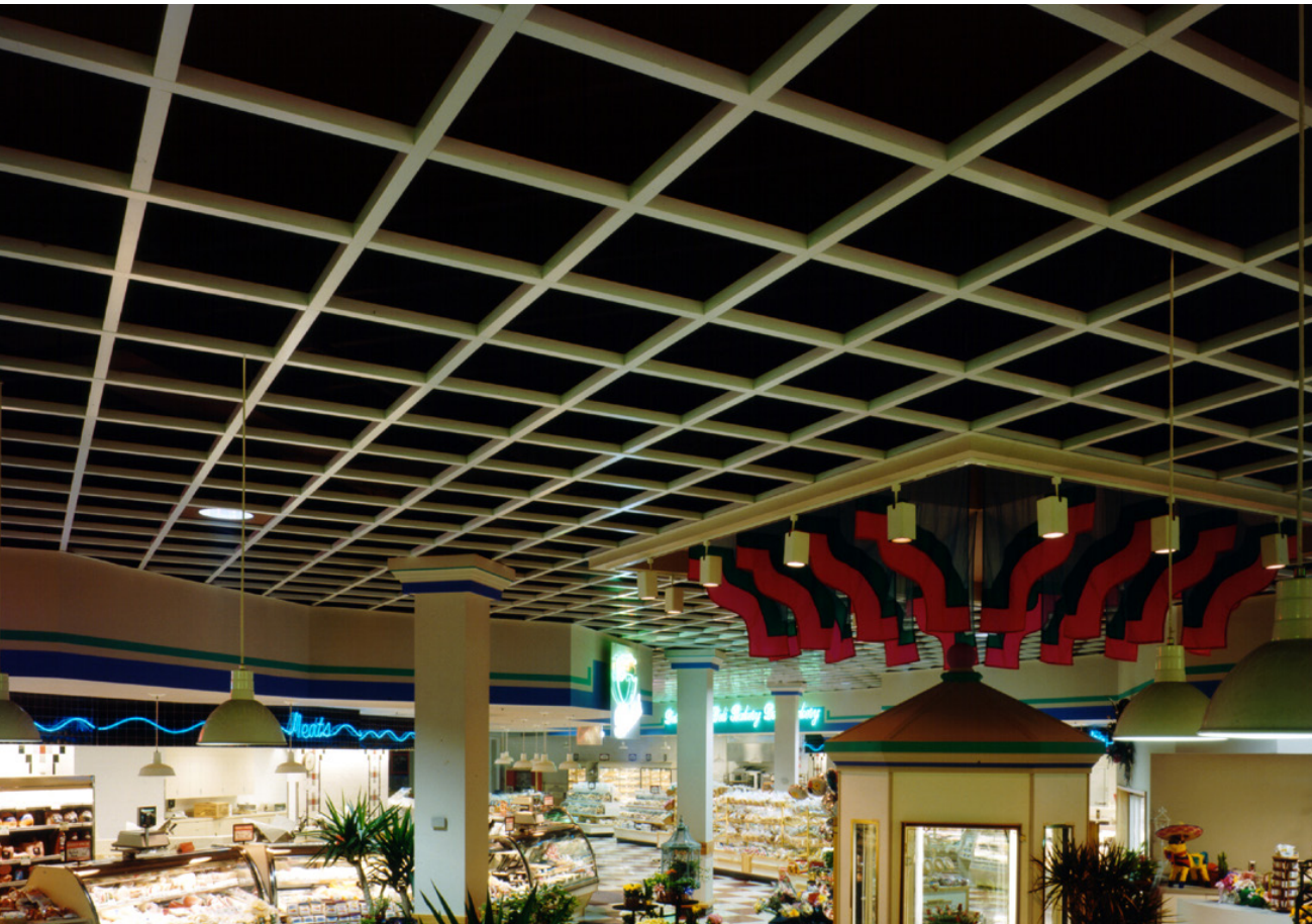
Project – Grocery Store Installation Product – Rockfon® Beamgrid®
